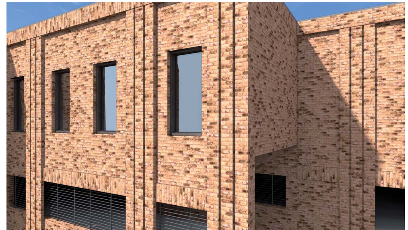
Front Elevation Close-Up View
